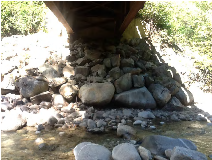
Right Bank Abutment when facing downstream
