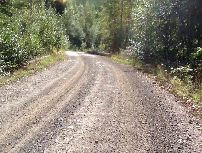
Right approach facing structure
