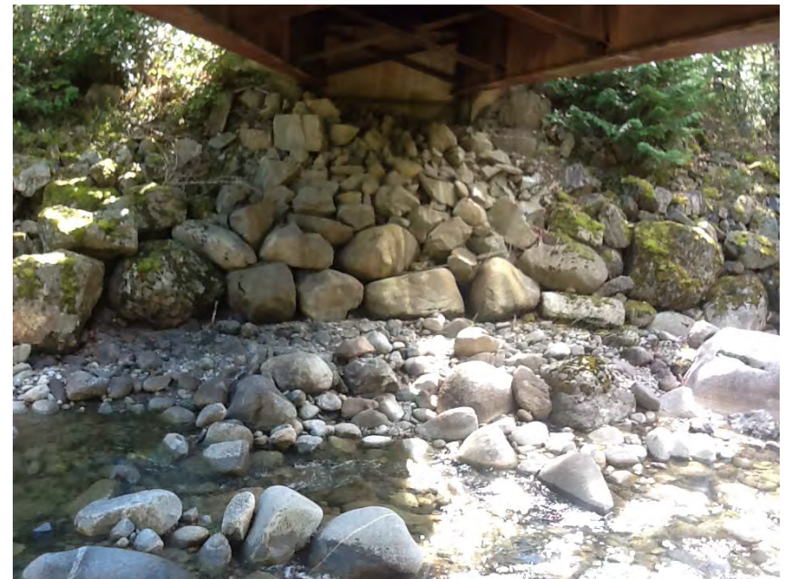
Left Bank Abutment when facing downstream
