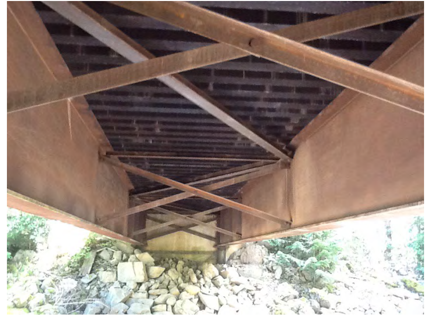
Underside of bridge
