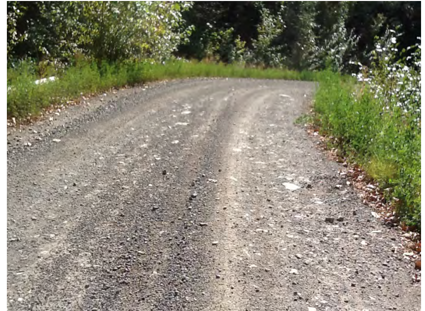
Left approach facing away from structure
